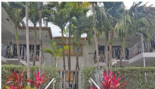
Apartment courtyard with geometric railing, Miami, FL
