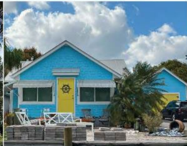
Stoop, window surrounds and wood shingles, Port Salerno, FL
