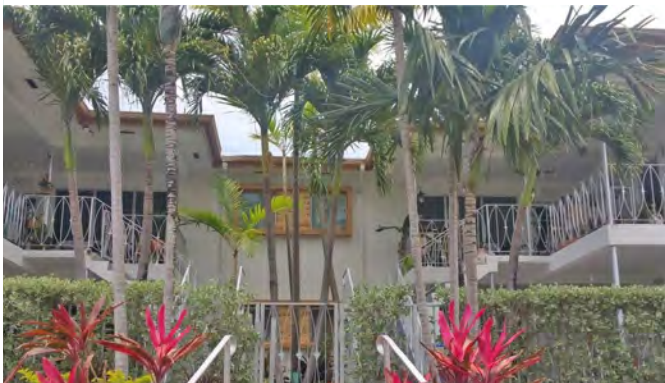
Apartment courtyard with geometric railing, Miami, FL
