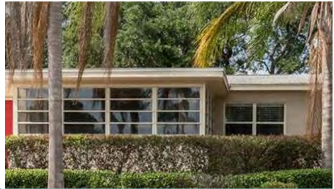
Large horizontal awning windows, Orlando, FL
