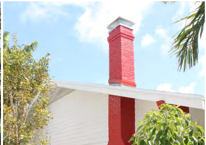
Brick chimney, West Palm Beach, FL
