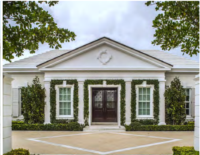
Georgian Residence. North Palm Beach, FL
