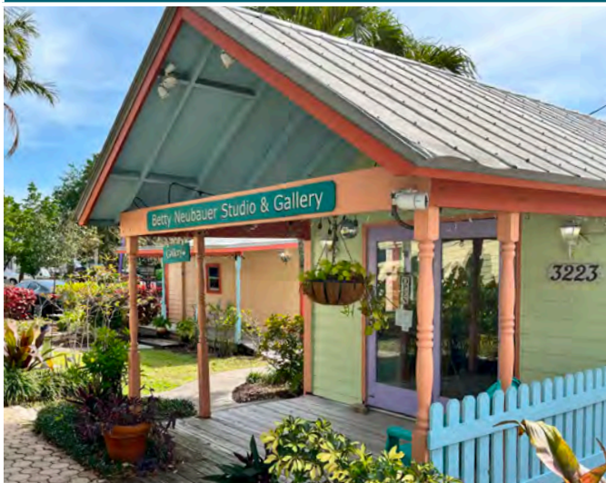
Porch and gable end at front of shop, Jensen Beach, FL
