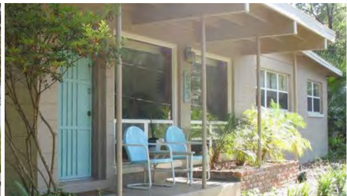
Pipe columns on a porch, Gainesville, FL
