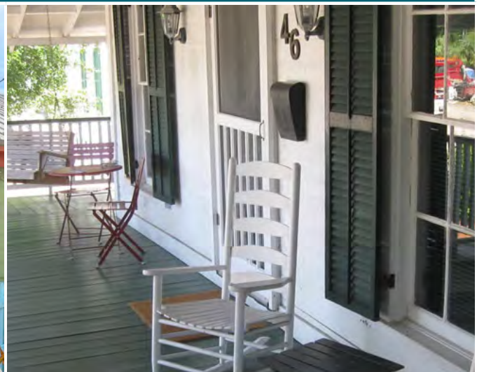
Wrap-around porch and operable shutters, Apalachicola, FL
