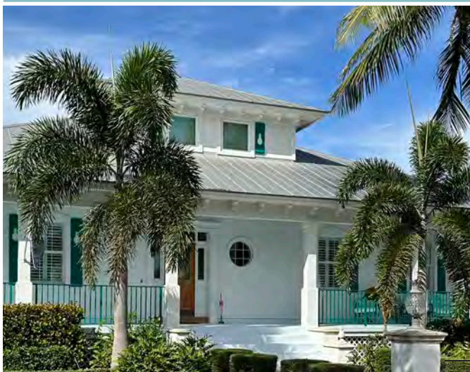
Dormer on hip roof and a wrap around porch, Hobe Sound, FL
