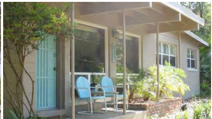
Pipe columns on a porch, Gainesville, FL
