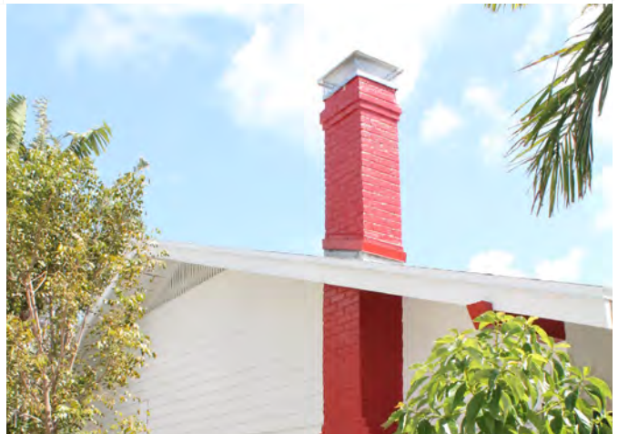
Brick chimney, West Palm Beach, FL
