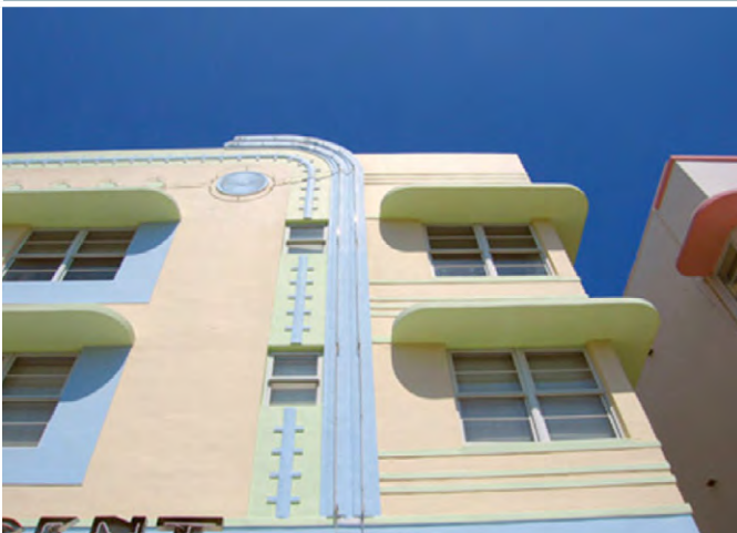
Vertical decorative facade treatment with rounded eyebrow at windows, Miami Beach, FL
