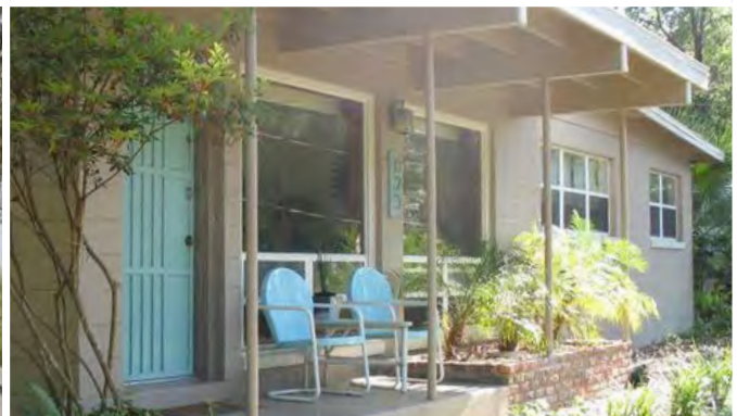
Pipe columns on a porch, Gainesville, FL
