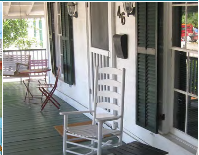
Wrap-around porch and operable shutters, Apalachicola, FL
