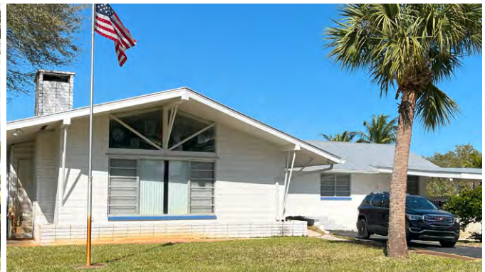
Gable roof with beams and pole brackets, Rio, FL
