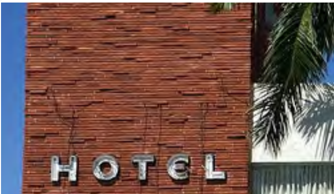
Brick facing with decorative signage. Miami, FL
