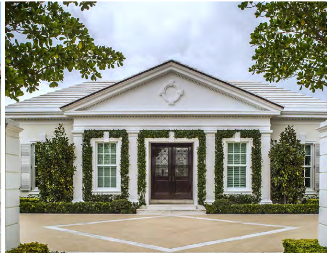
Georgian Residence. North Palm Beach, FL
