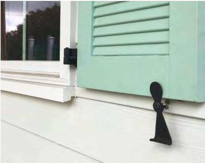
Detail of an operable shutter and shutter stay
