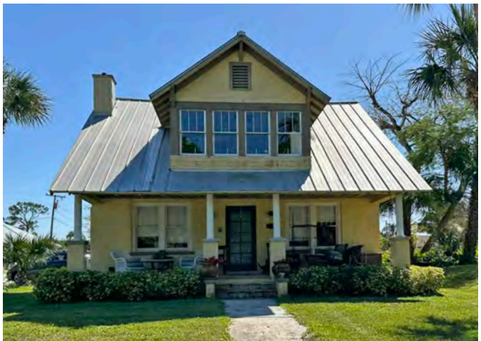
Larger dormer with shingle siding and 3 over 1 double-hung windows, Old Palm City, FL
