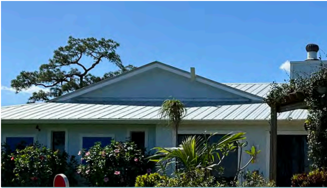
Low-slope roof with Dutch Gable roof detailing and rectangular chimney, Old Palm City, FL
