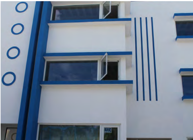
Fixed glass casement window, West Palm Beach, FL
