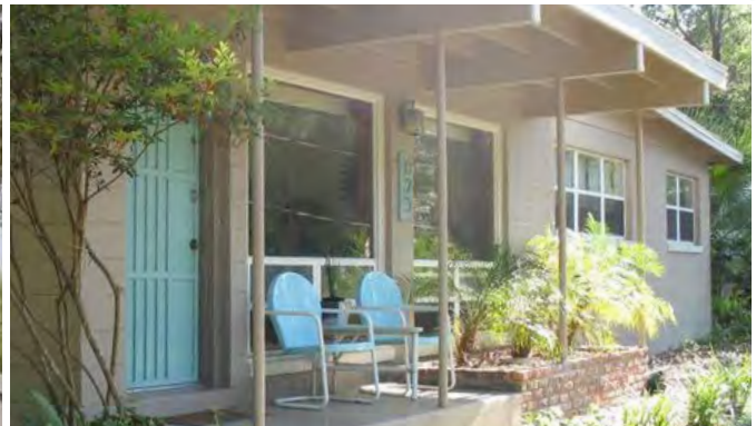
Pipe columns on a porch, Gainesville, FL
