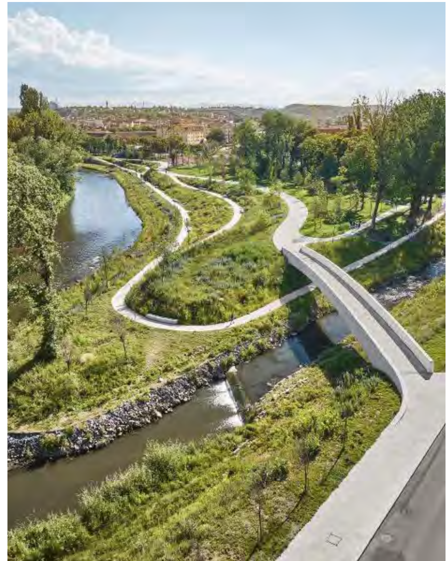
RIVER SOMES PARK, CLUJ-NAPOCA, ROMANIA TRAIL & FOOTBRIDGE
