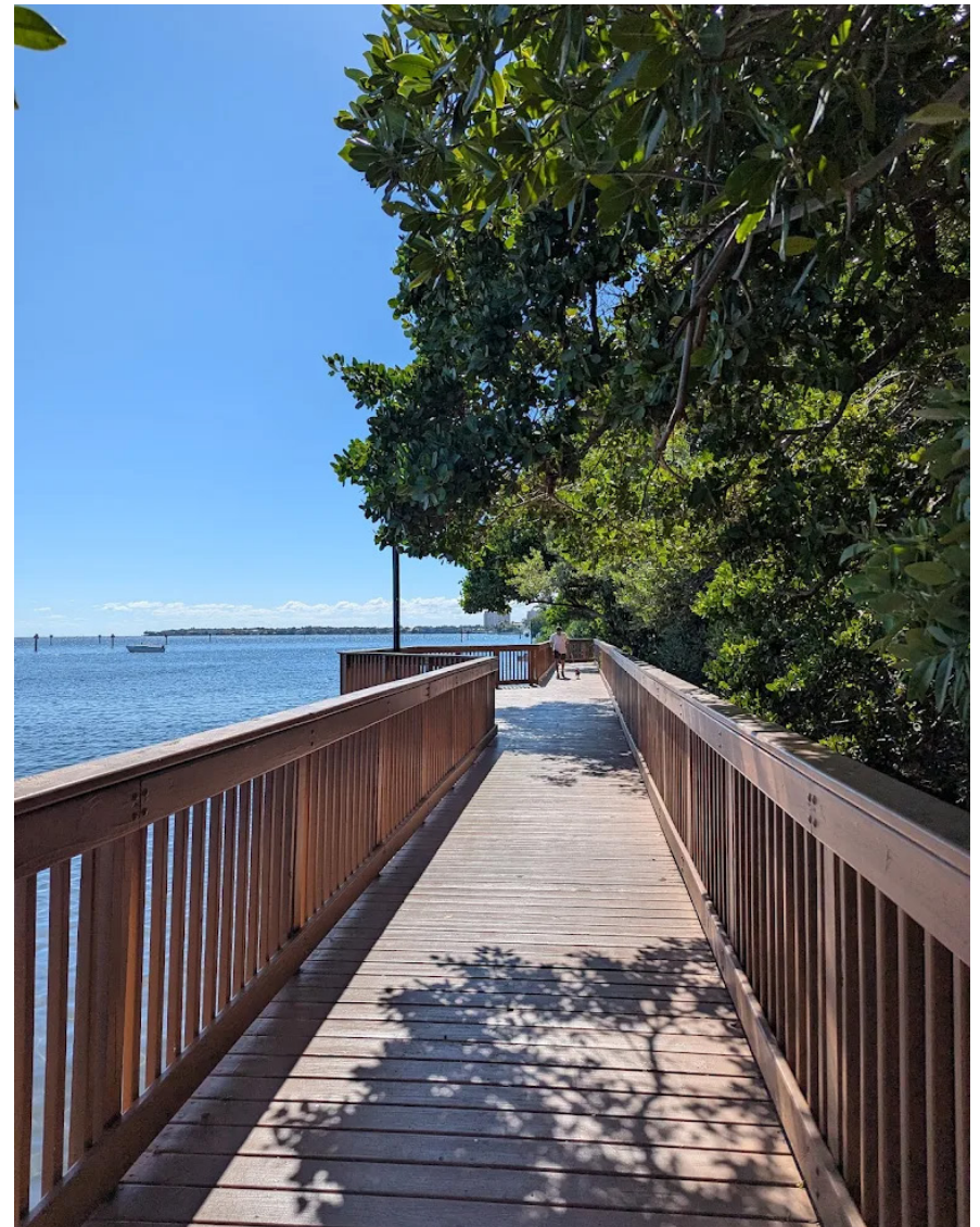
PEACOCK PARK, COCONUT GROVE, MIAMI-DADE COUNTY BOARDWALK ON THE WATER
