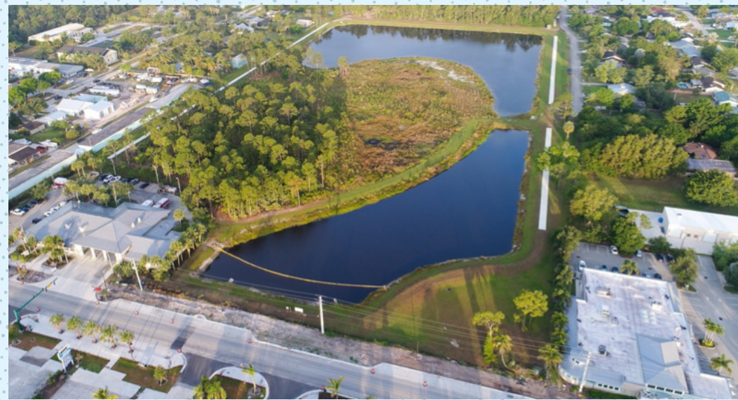
Mapp Road in the Old Palm City CRA - the 2021 Florida Redevelopment Association's "Capital Project/Infrastructure" award winner!
