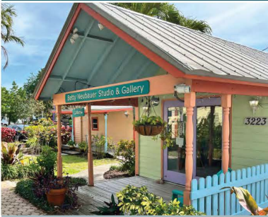
Porch and gable end at front of shop, Jensen Beach, FL
