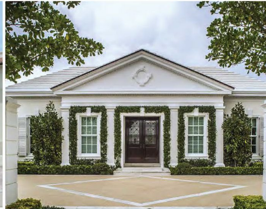
Georgian Residence. North Palm Beach, FL
