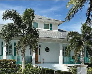
Dormer on hip roof and a wrap around porch, Hobe Sound, FL
