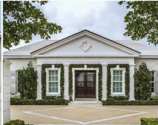
Georgian Residence, North Palm Beach, FL
