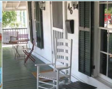
Wrap-around porch and operable shutters, Apalachicola, FL
