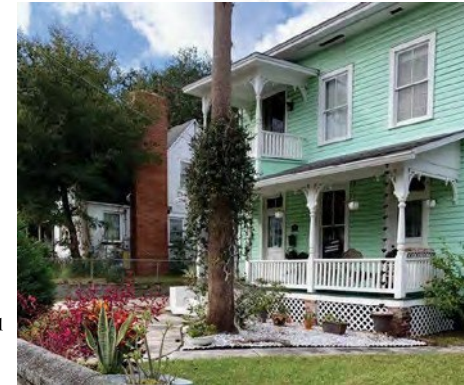
Piers with latticework. Image by ML+H.
