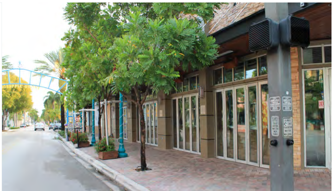
Operable glass wall as part of storefront, Delray Beach, FL
