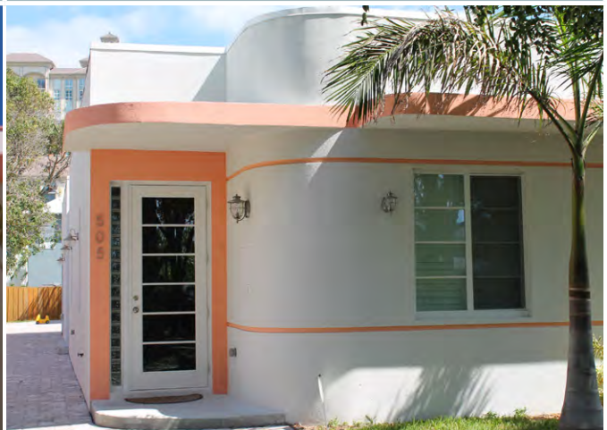
Smooth stucco walls and windows/door with horizontal lights, West Palm Beach, FL
