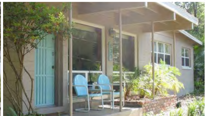
Pipe columns on a porch, Gainesville, FL
