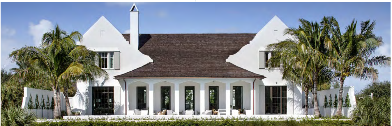
House in Windsor, FL by Moor Baker Architects photographed by Jessica Glynn
