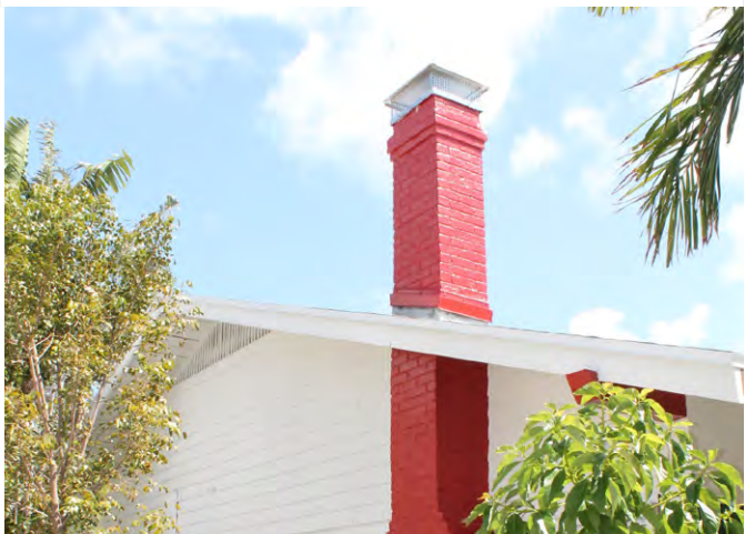
Brick chimney, West Palm Beach, FL
