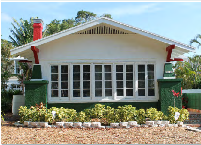
A Bungalow with a bank of casement windows, West Palm Beach, FL
