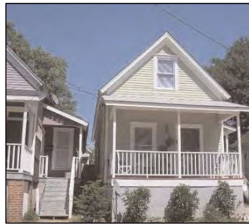
SHOTGUN HOUSE, SAVANNAH, GA: The shotgun typology (long and narrow with front porch) is a simple example of Florida's wood vernacular style. The components are a raised base, covered porch, gable end facade and simple wood moldings around the doors and windows.
