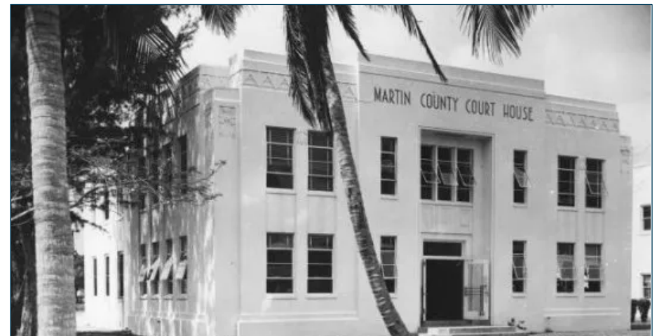
MARTIN COUNTY COURTHOUSE, 1923
