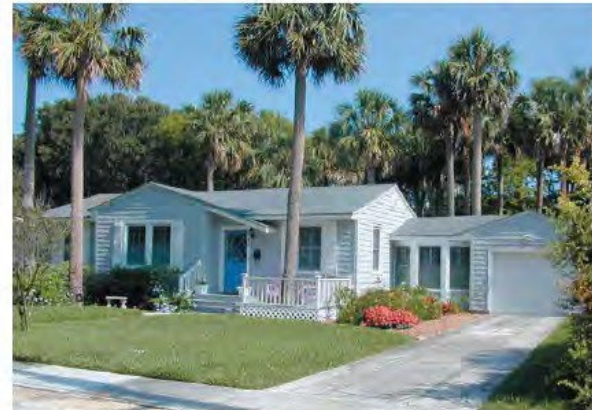
Positioning the garage behind the front wall plane lessens its visual impact.
