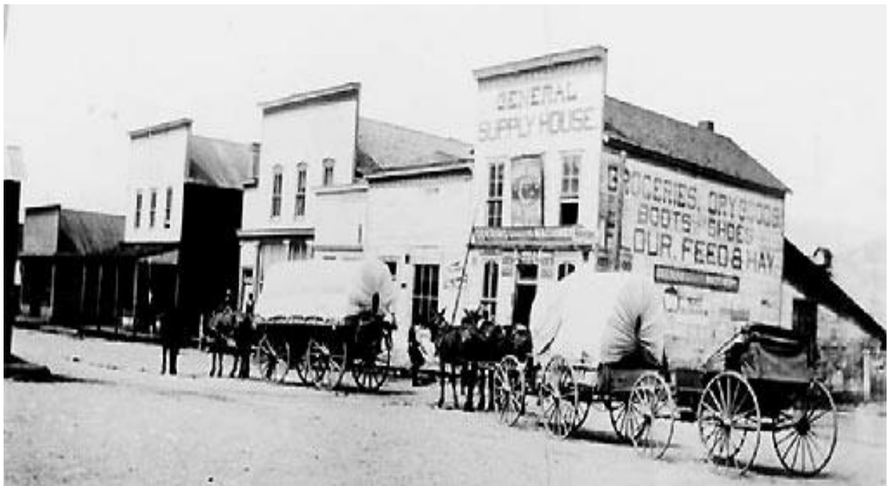
FIGURE 50. FALSE FRONT WOOD FRAME COMMERCIAL BUILDINGS COLORADO
