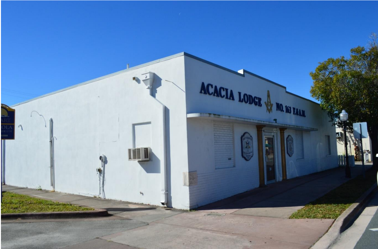
FIGURE 46. ACADIA LODGE, 14 SE OSCEOLA STREET
