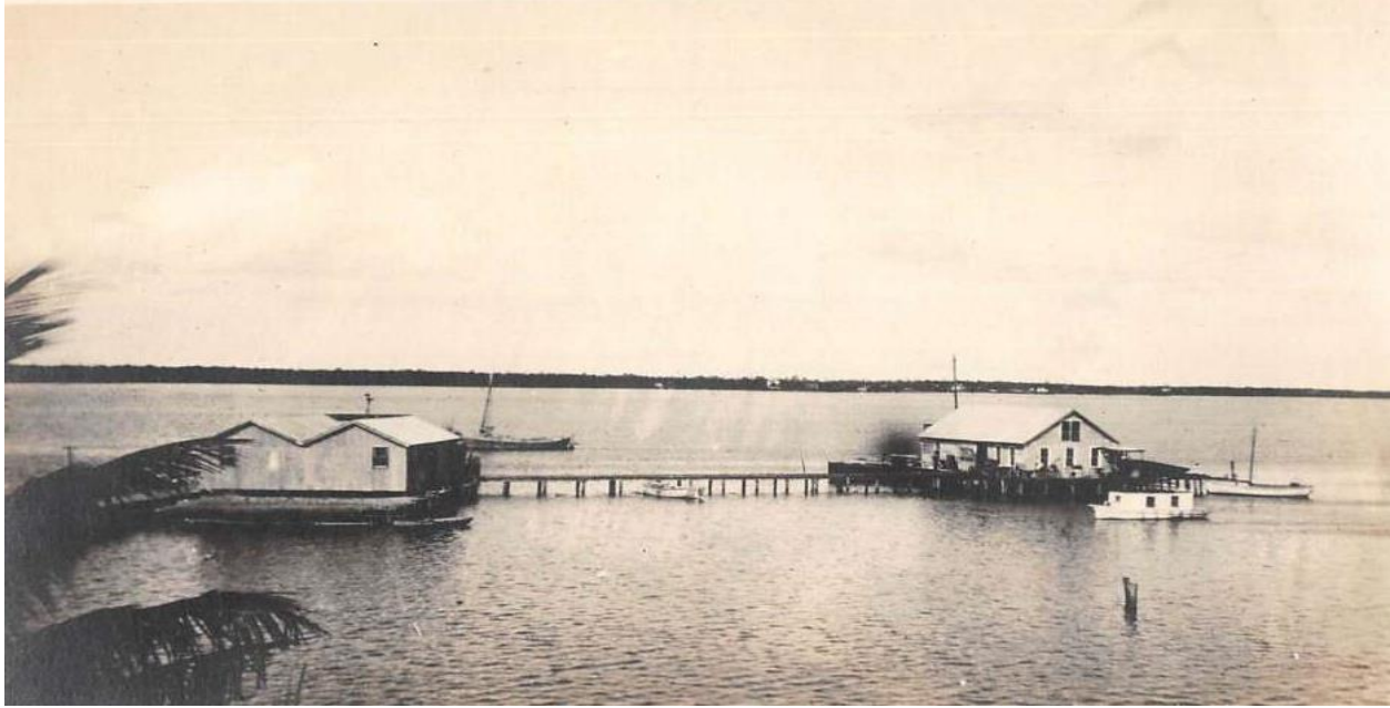
FIGURE 9. STUART'S FIRST FISH HOUSE SOUTH SIDE RAILROAD BRIDGE, C. 1895
