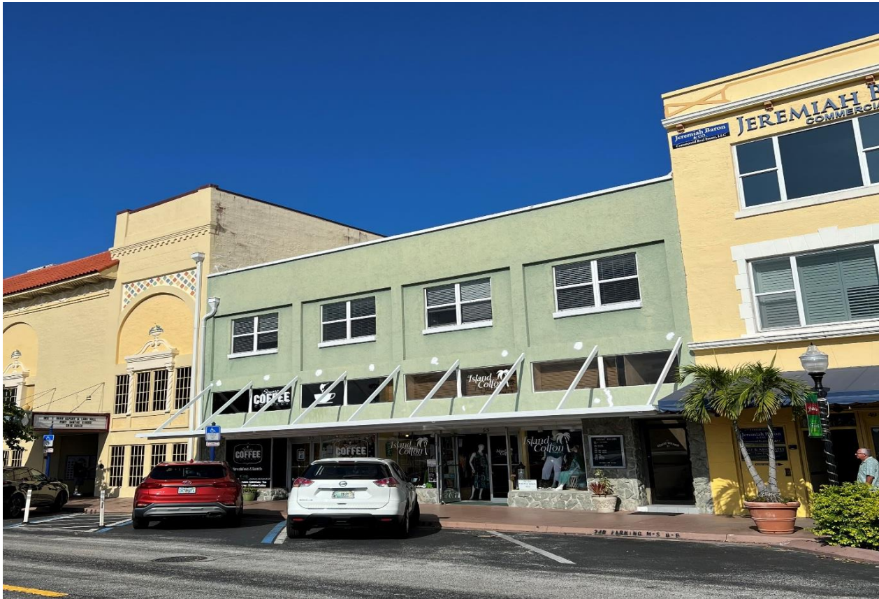
FIGURE 55. GREEN BUILDING 51 SW FLAGLE AVENUE
