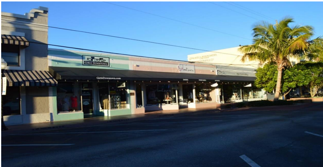
FIGURE 51-52. 27-29 FLAGLER AND PRESSEL BUILDING FLAGLER AVENUE
