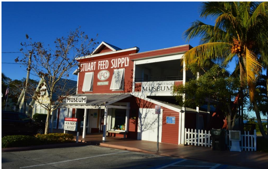
FIGURE 48. STUART FEED STORE, FALSE FRONT COMMERCIAL BLDG.
