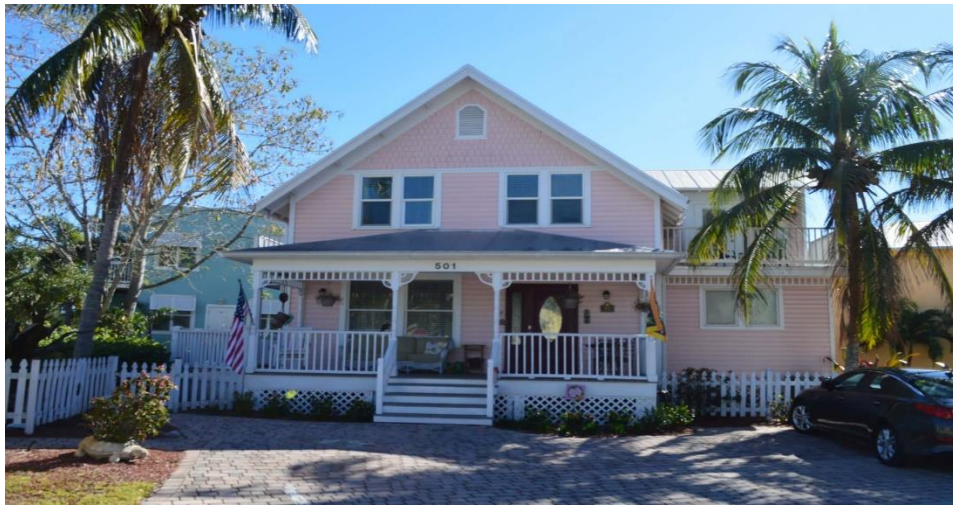
FIGURE 56. SAM MATHEWS HOUSE, 501 AKRON AVENUE
