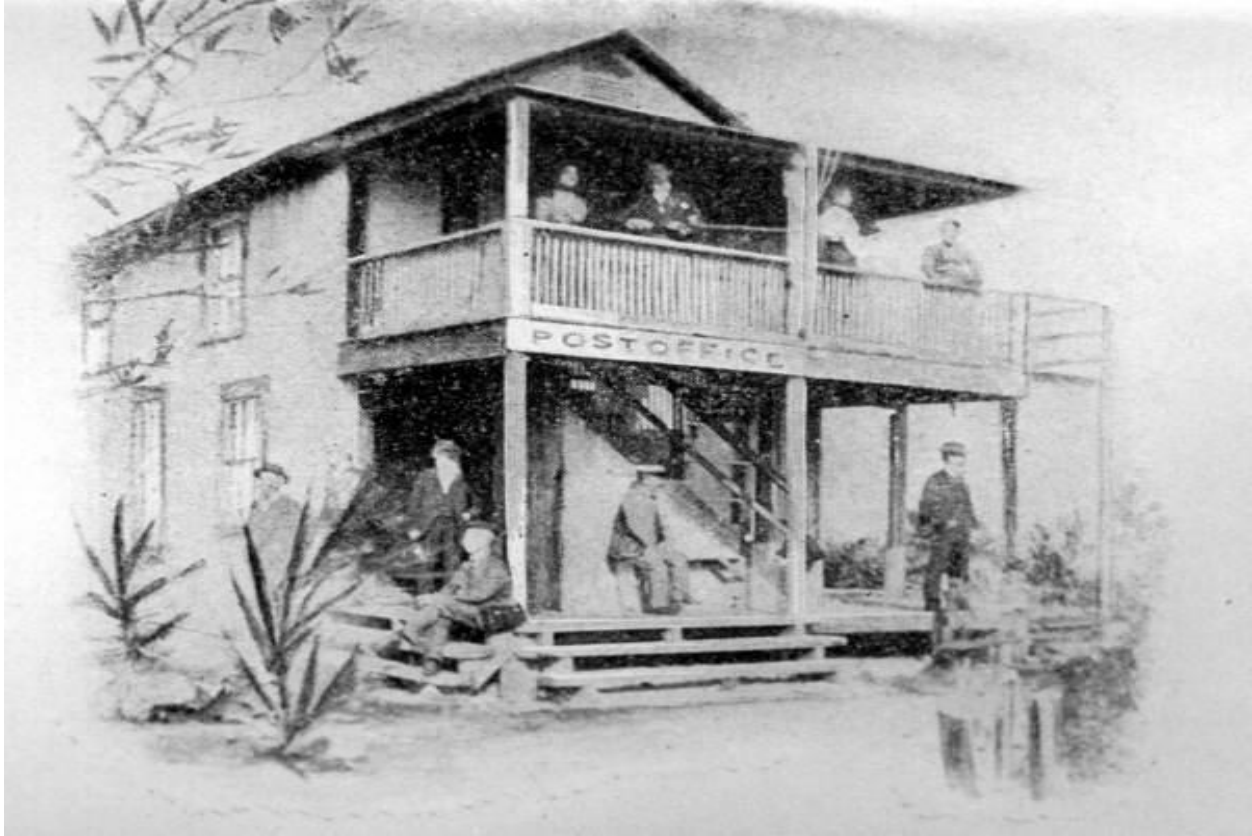
FIGURE 7. WALTER KITCHING STORE AND STUART POST OFFICE, C. 1895
