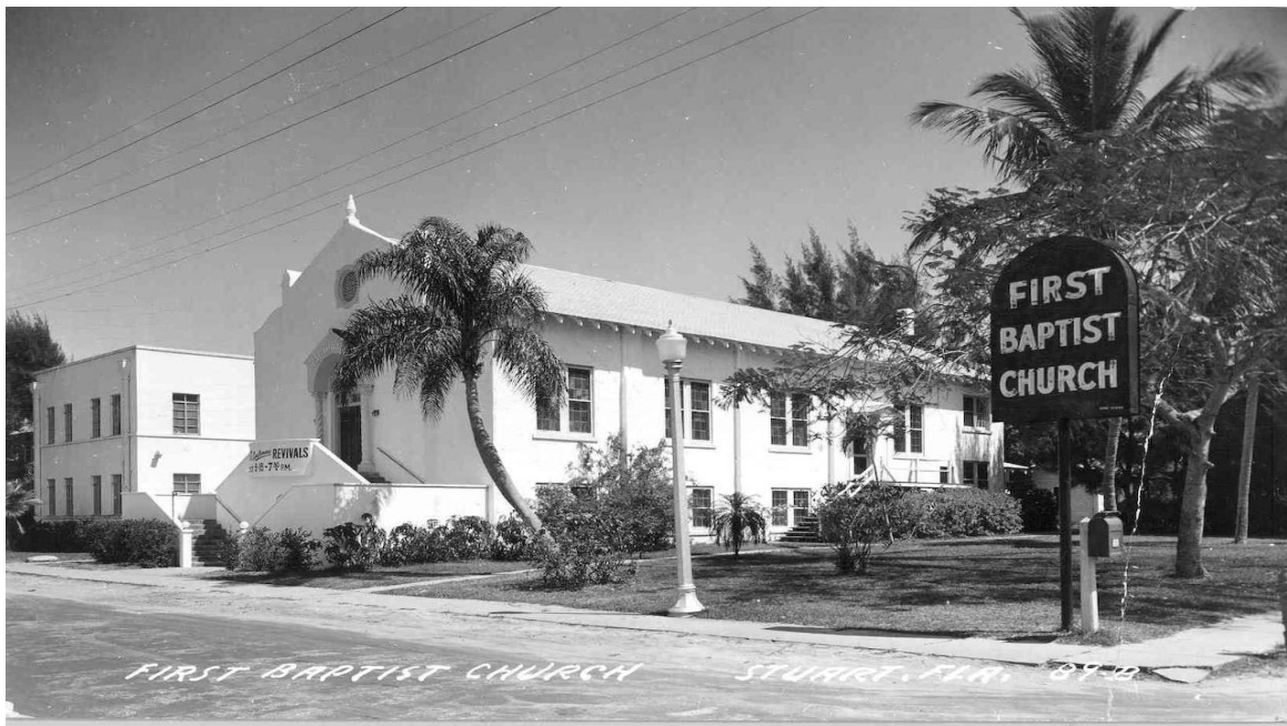
FIGURE 21. FIRST BAPTIST CHURCH, 200 SW AKRON AVE, NOW DEMOLISHED
