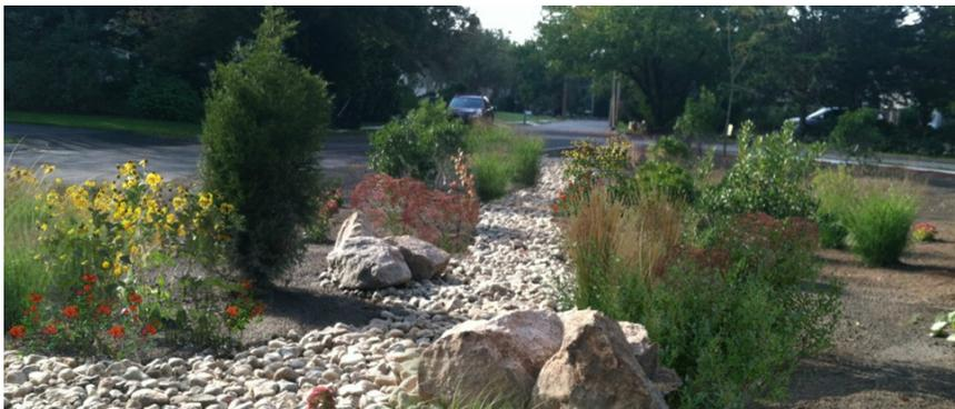
*"Bioswales are stormwater runoff conveyance systems that provide an alternative to storm sewers. They can absorb low flows or carry runoff from heavy rains to storm sewer inlets or directly to surface waters. Bioswales improve water quality by infiltrating the first flush of stormwater runoff and filtering the large storm flows they convey."*
